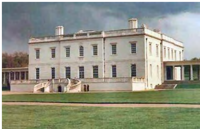
The Queens House. A.Palmer, Greenwich Guide
